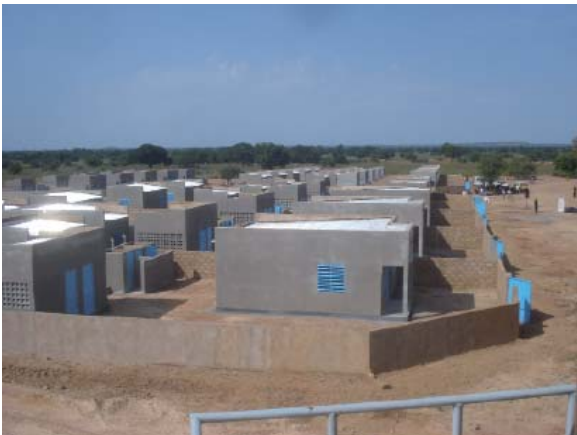
28 completed houses and associated facilities
