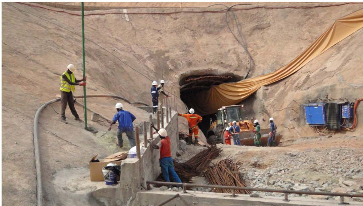
Underground Mine Portal Entrance
