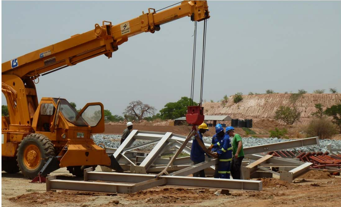
Assembling Steel Framework
