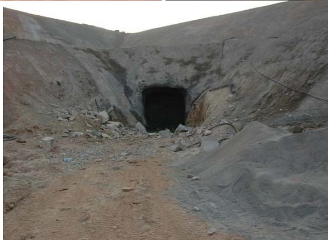
Development of decline commenced on 16 May 2008 following first blast.
