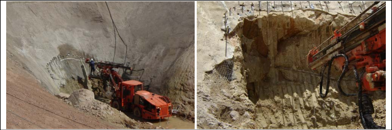
Sandvik drilling 'jumbo' preparing site of portal for excavation
