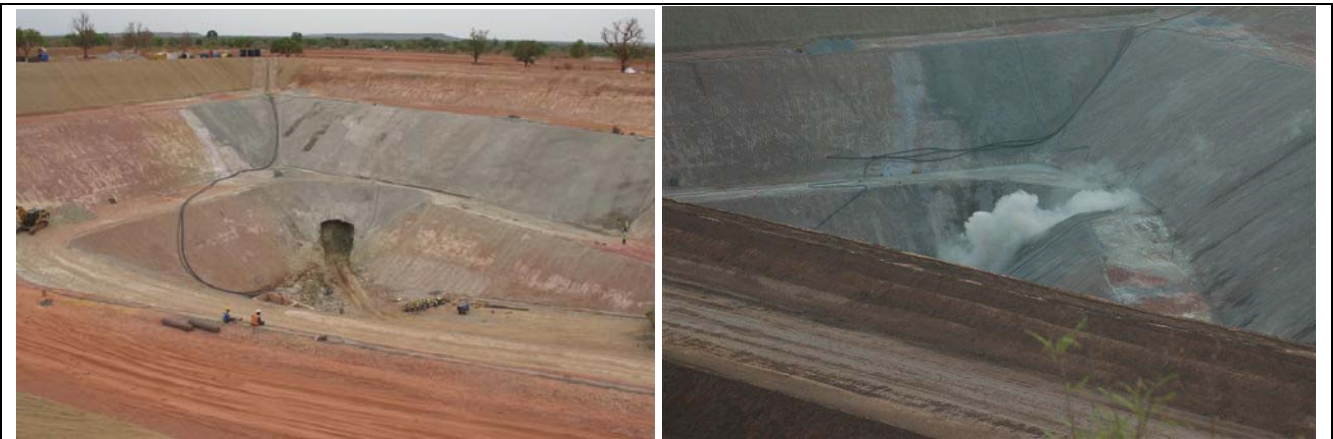
Initial excavation of portal commenced using Caterpillar underground loader
