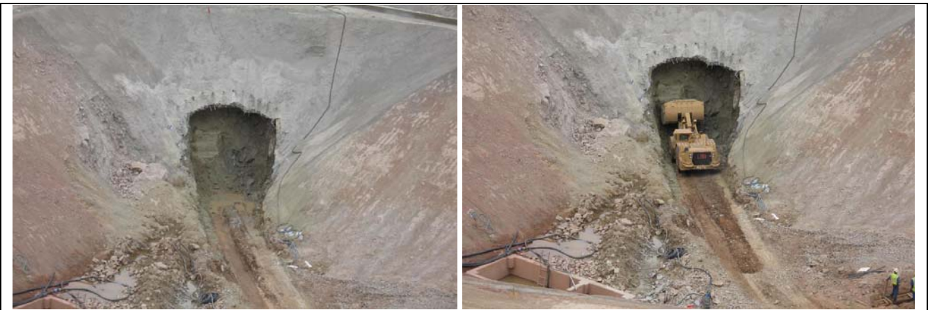
Initial excavation of portal commenced using Caterpillar underground loader
