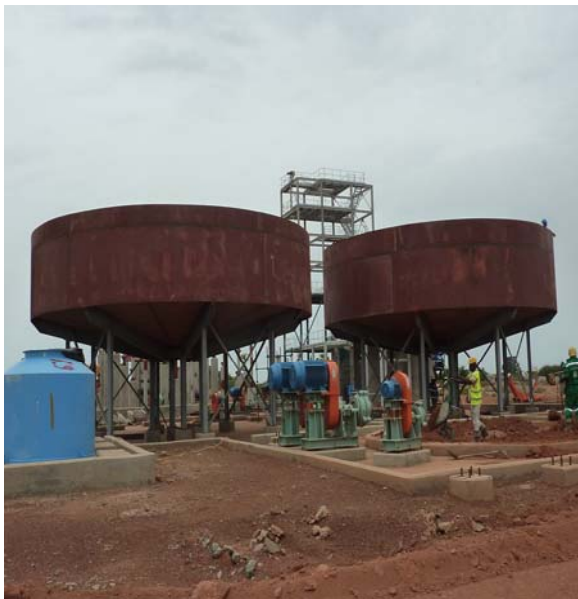
Perkoa Plant Construction
