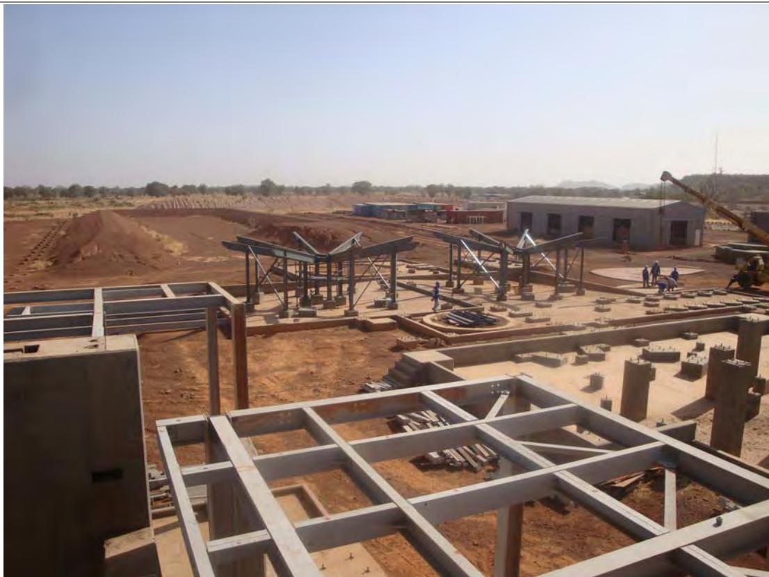
On-site construction continues Photo taken: 6/2/2010
