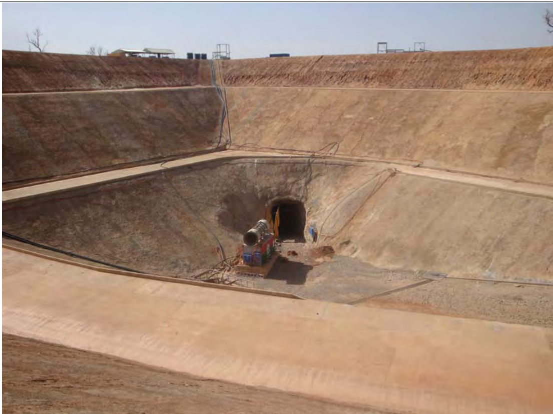
Box-cut and portal Photo taken: 4/2/2010
