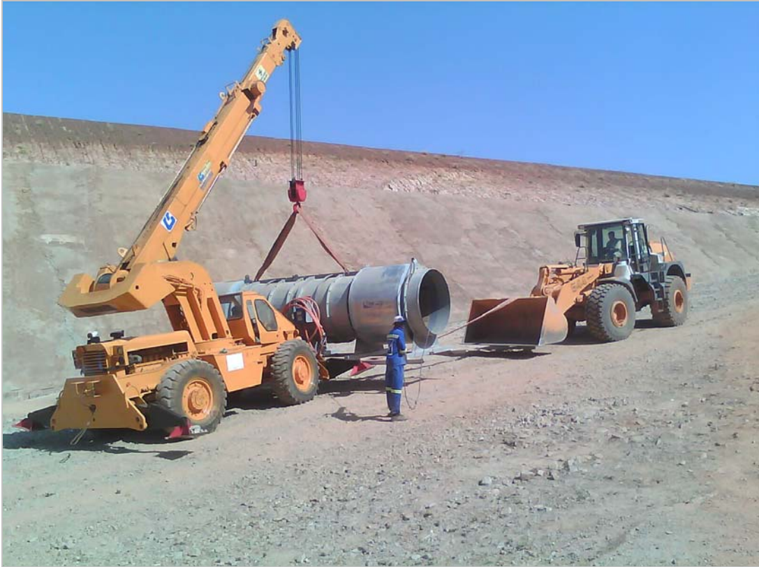
FIGURE 1 - Photograph showing work in progress at Perkoa including maintenance of mine ventilation system.
